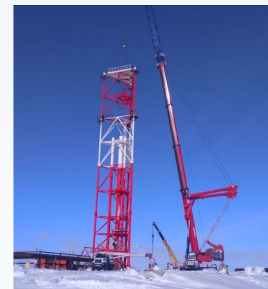
Combined Forced-Air Flare System
